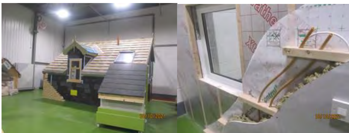
Photos: Mock house to demonstrate air tightness, Enniscorthy retrofit training centre
