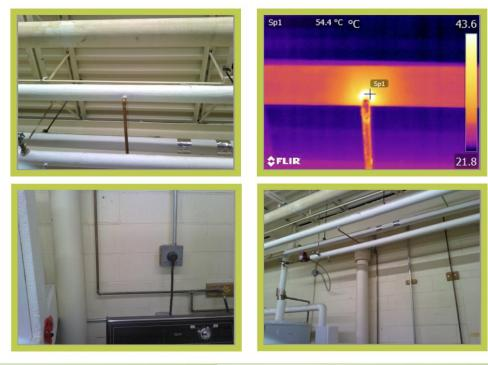
Operating Temperature, \*F122Ambient Temperature, \*F75Insulation selectedFiberglass
